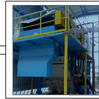
Coolant Recycle System Capacity -30KLD
